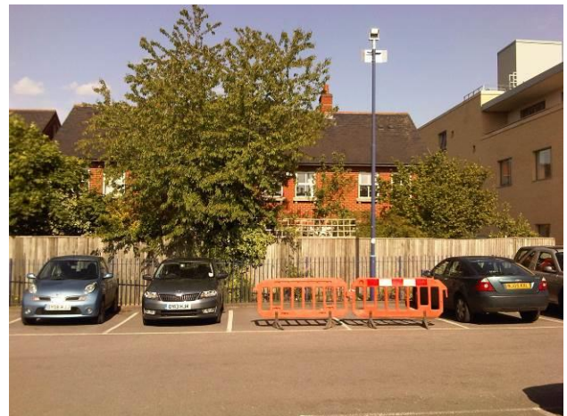
Boundary fence between Network Rail land & the Stable Close properties
